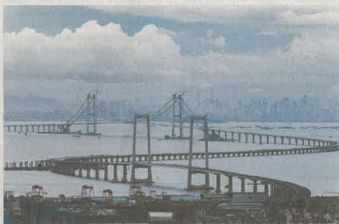
The Shenzhen-Zhongshan bridge is part of a cross-sea span that will boost economic integration in the Greater Bay Area. Photo: Getty Images
